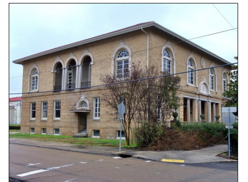
The Prentiss Club after restoration of the roof, cornice, windows, side entrance canopy,
