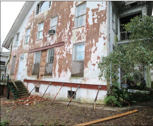
Stabilization work at Melmont is visible on the exterior and interior, where frame stud walls have now been built within the brick walls to support the house while the brick walls are repaired or rebuilt as necessary.
